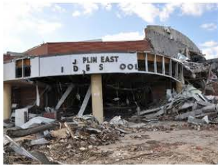
Building Damage and Surroundings
